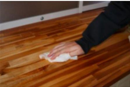
9. In order to ensure 100% uniform and smooth finish, just DRU BUFF the surface using a clean wool pad (or cotton cloth under the orbital sander) to dry polish mechanically
