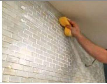
Once the grout is set and dry and if there is still residue use nylon brush to clean and then apply grout sealer according to manufacturer's instructions.
