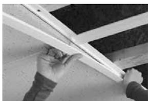
**Surface Mount Grid System** - CeilingMAX® is engineered for direct application over plaster, drywall and glue-up ceilings. This surface-mounted grid system saves up to 6" of ceiling height.
