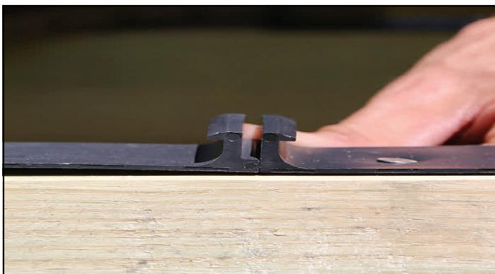
Interlock clip strips along each joist and fasten with roofing nails.
