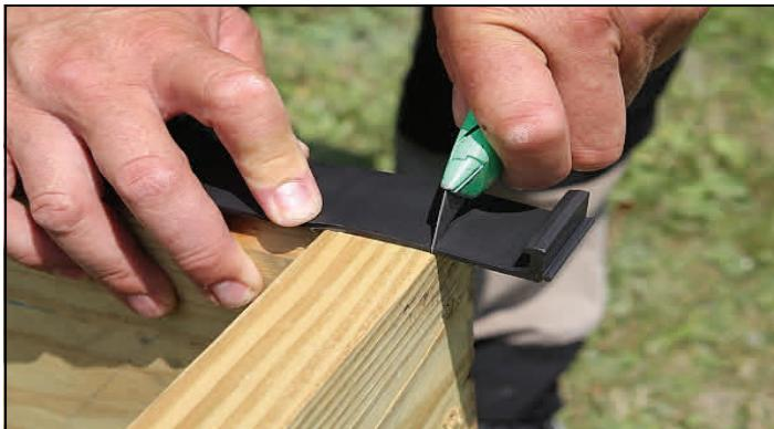
Score and trim each clip strip flush with the outer edge of the rim joist to facilitate Starter board installation.
